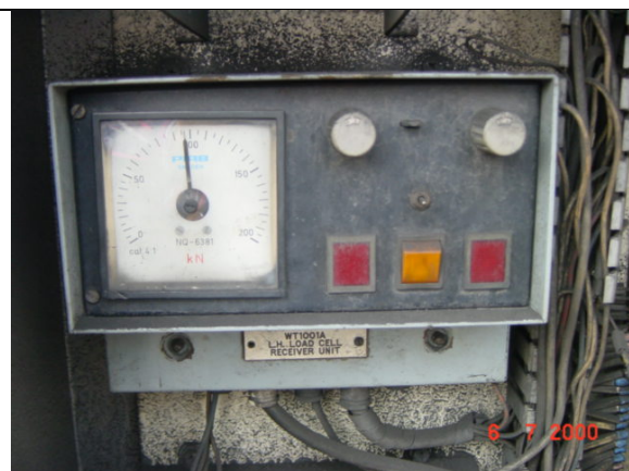
Photo X. PIAB ARLL Analogue Readout Load Limiter (6:64) enabling continuous analogue readout of the conveyor belt tension and two alarm settings, easily changeable by an potentiometer each. Overload immediately leads to a visual alarm.
